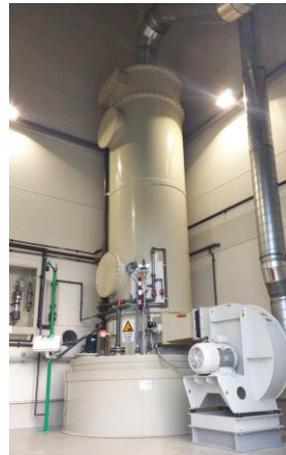
Fig. 1: chem. absorption scrubber for odour reduction 10.00  $\text{Bm}^3/\text{h}$
