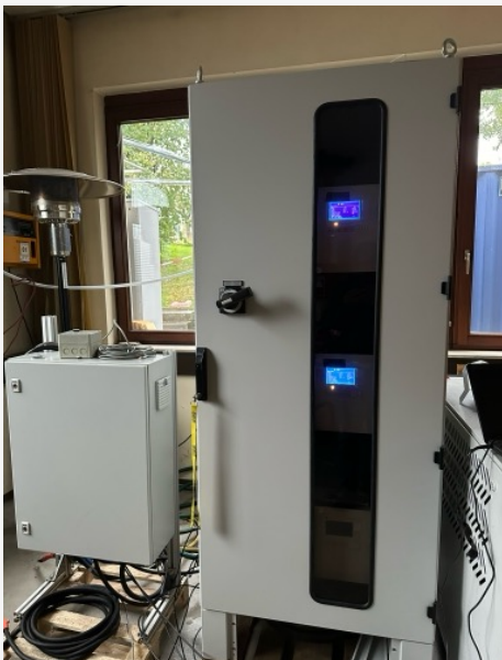
Power supply with 120 kW, modular setup
